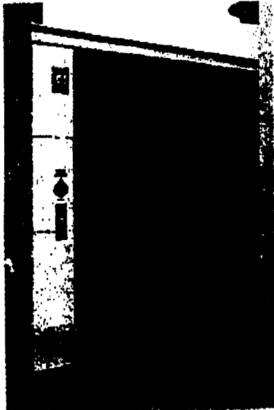
Deployed Smoke Guard System
