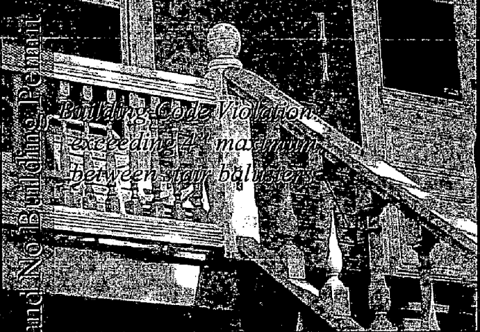
Newel Post lacking adequate detailing
