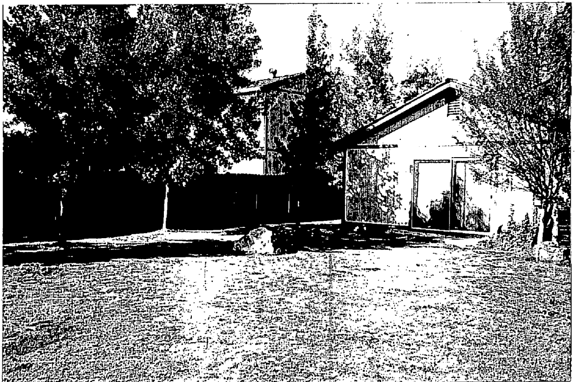
Fig. 6. Looking across the installation site to the West, the row of liquidambar trees is sufficient to completely screen the nested tower.
