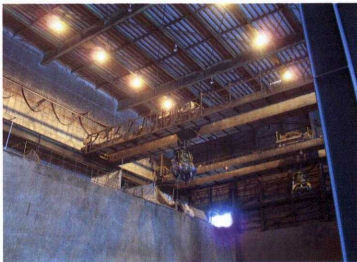
Figure 3 Solid waste lifted to shredder
