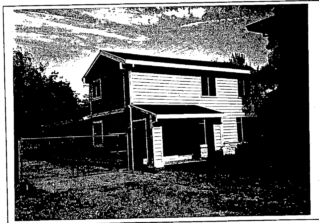
view of existing house which is currently under renovation
